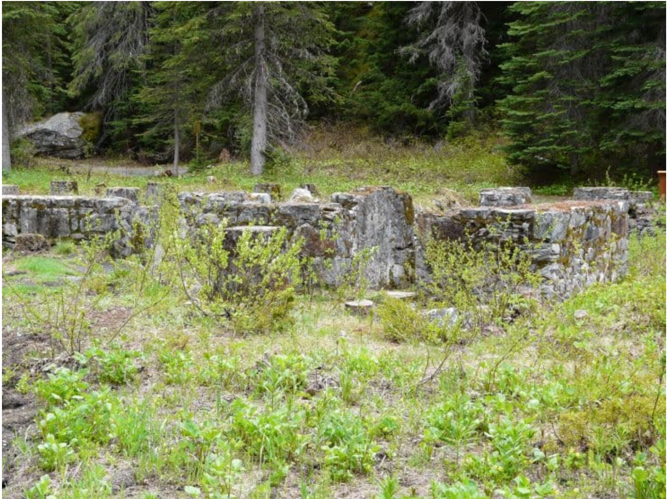
Fundamente Glacier House.JPG - Redonebird - https://creativecommons.org/licenses/by-sa/3.0/de/deed.en
